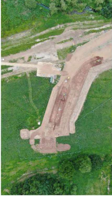
Aerial view of the West Tie in point
